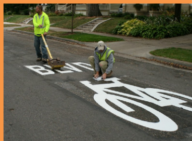
Above: Installing pavement markings (August 2011, Leslie Foreman) Right: A Bicyclist using the new experimental green shared lanes on Bryant (Sept 2011, TLC)
